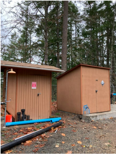
S03 under construction
