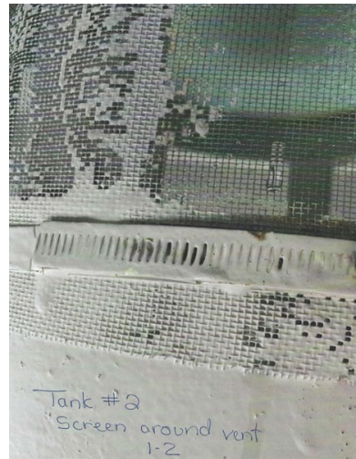
Reservoir #2 vent screened
