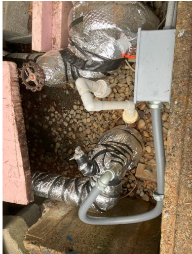
Well #1's vault, disconnected
